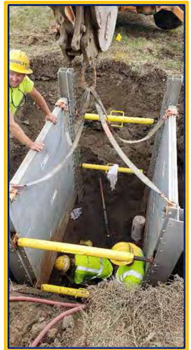
A Corning ops line crew works in a trench box.
